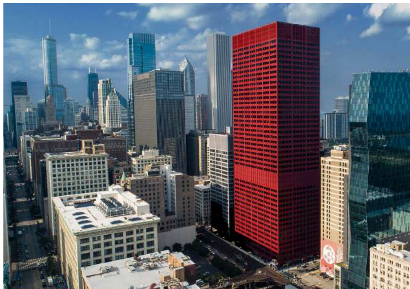
„BIG RED“ PRIME OFFICE TOWER – CHICAGO
